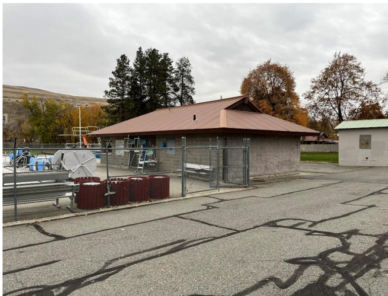
Plate 16 – Asphalt Cracking
