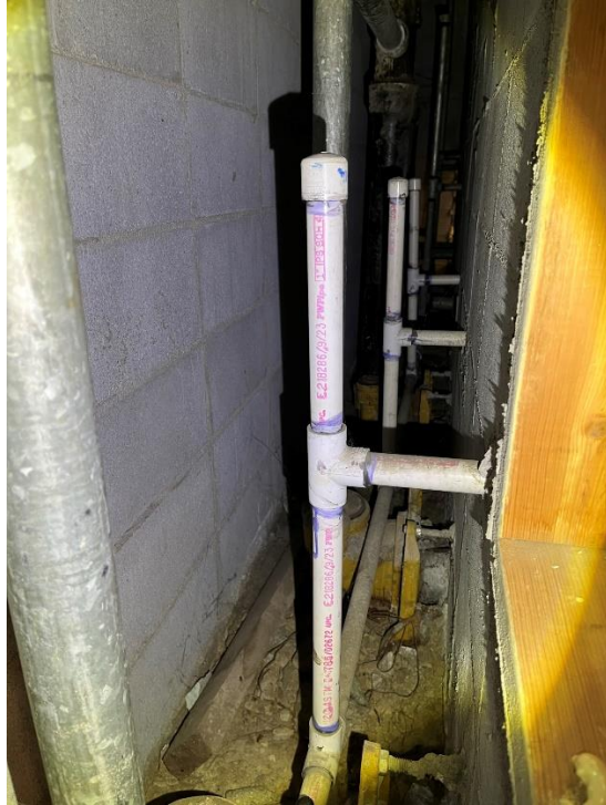
Plate 13 – Men's Restroom Wall Chase
